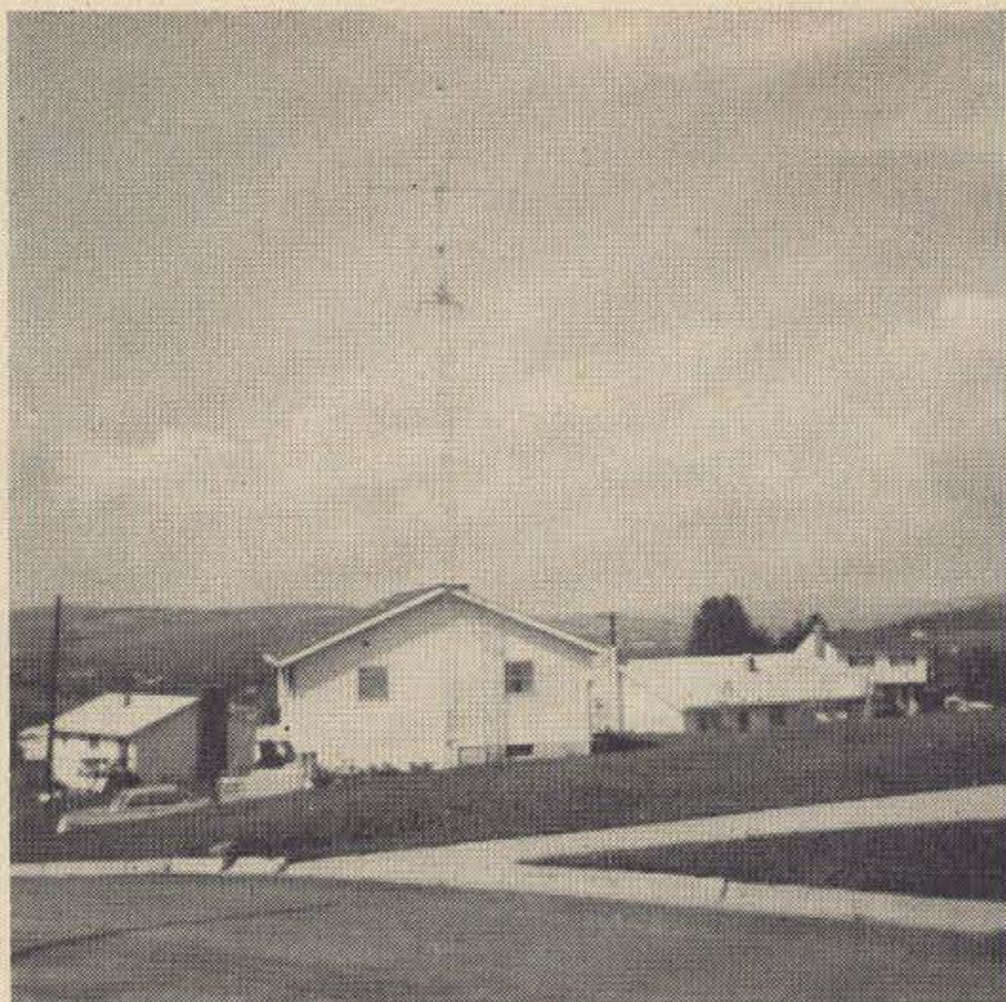
The erect tower—A neat installation
